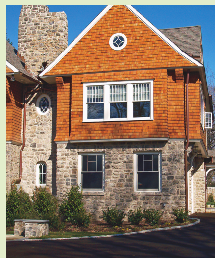
Gardner/Fox Associates reused the stone from the original arched entryway (left) to construct part of the two-and-a-half car garage addition (right).
